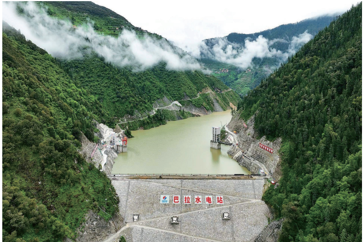
Figure 1: Bala Hydropower Station
